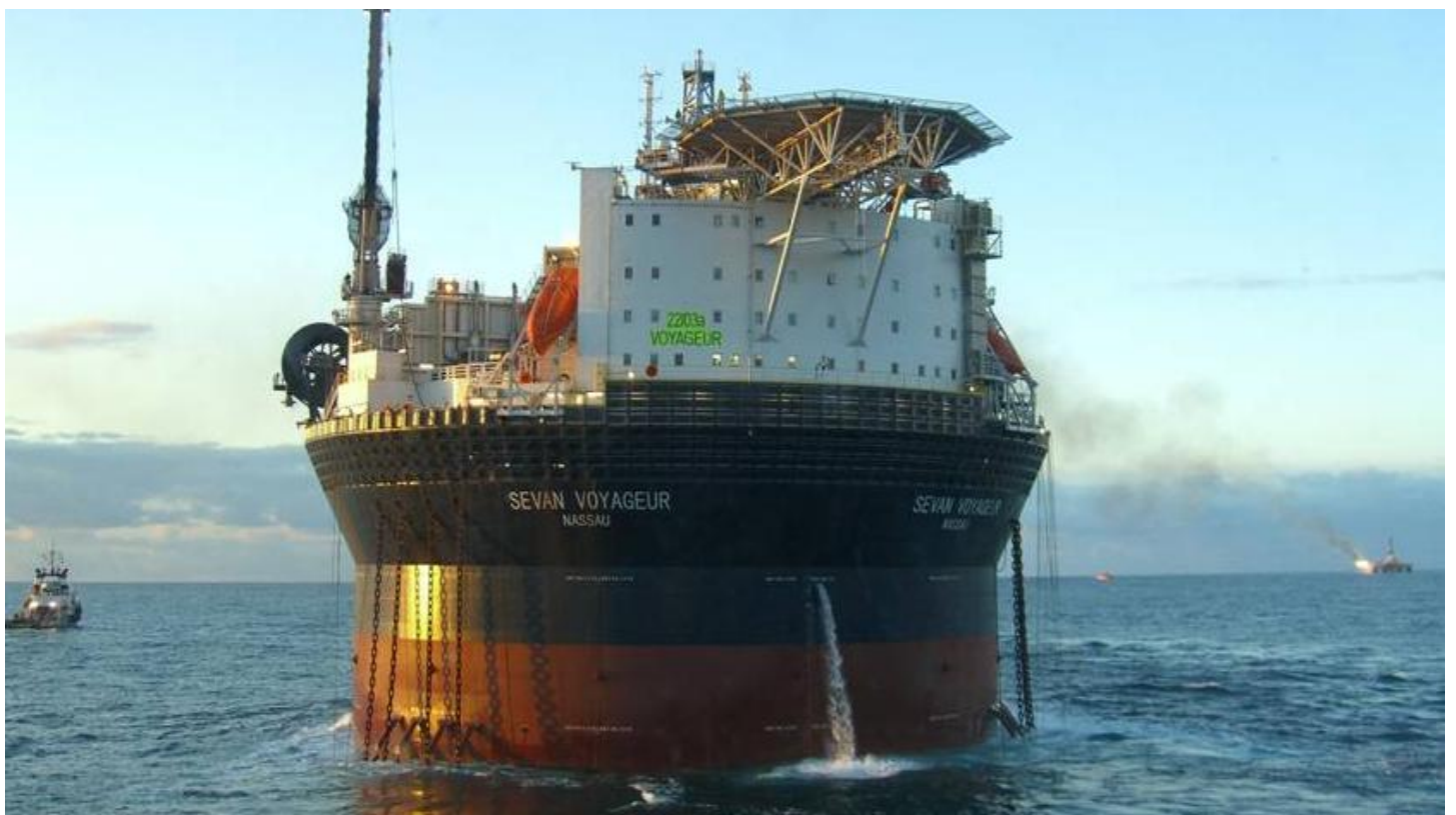
FPSO Sevan Voyageur at the Shelley field in the UK Central North Sea
