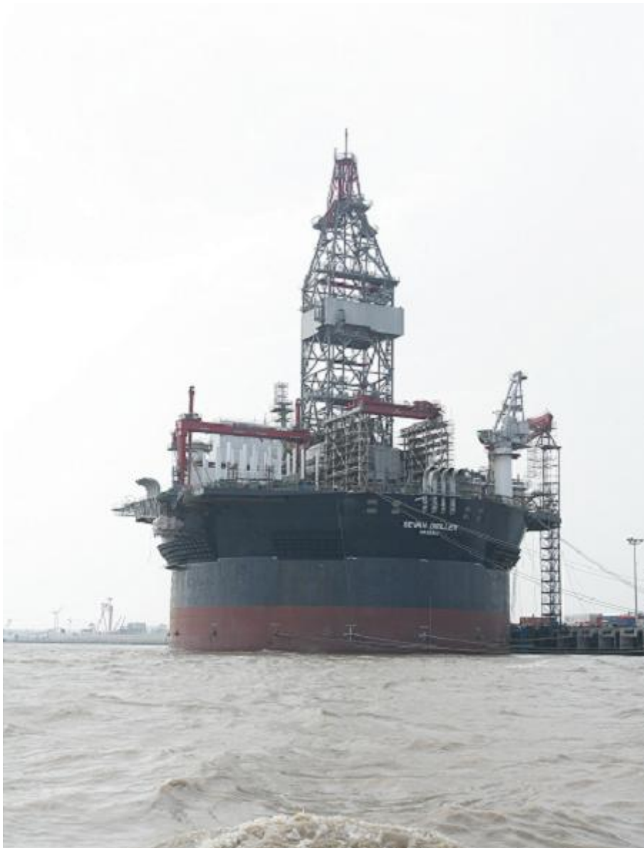
April 2009 - Sevan Driller at COSCO Qidong Shipyard
